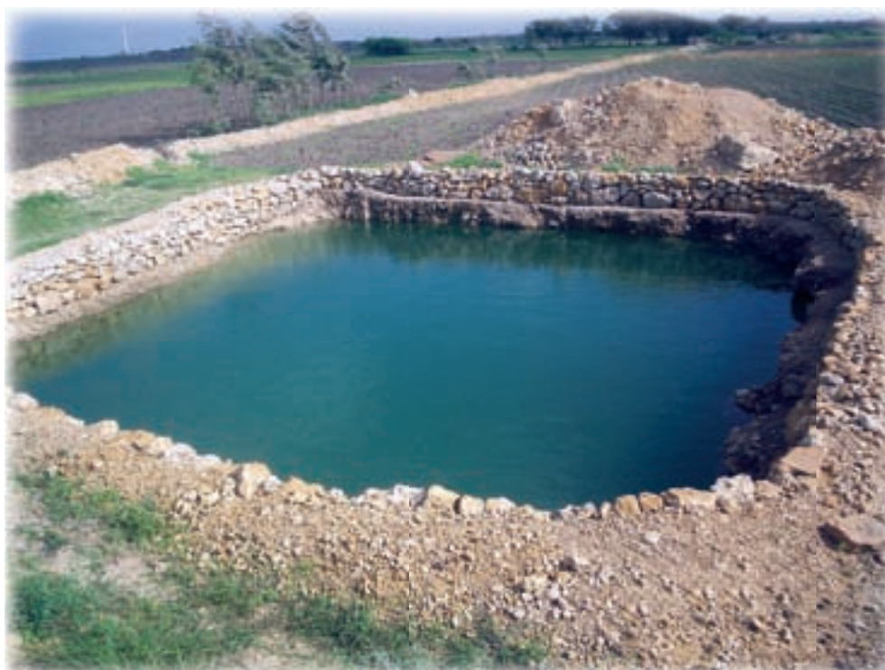
Kharash Vistarotthan Yojana (KVY): Promotion of farm ponds for retention of water by the Coastal Salinity Prevention Cell (CSPC) in Sattapar village, Jamnagar district, Gujarat.
