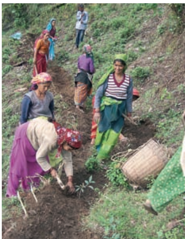
Himmothan Pariyojana: Trenching and planting being undertaken on steep slopes in Gadora village, Chamoli district, Uttarakhand under Himmothan's Integrated Fodder – Livestock Development Project.
